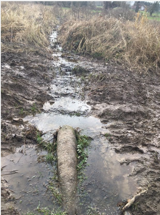
Location where the newly restored watercourse will come.
